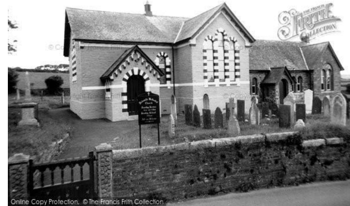
Dobwalls Chapel c.1965
